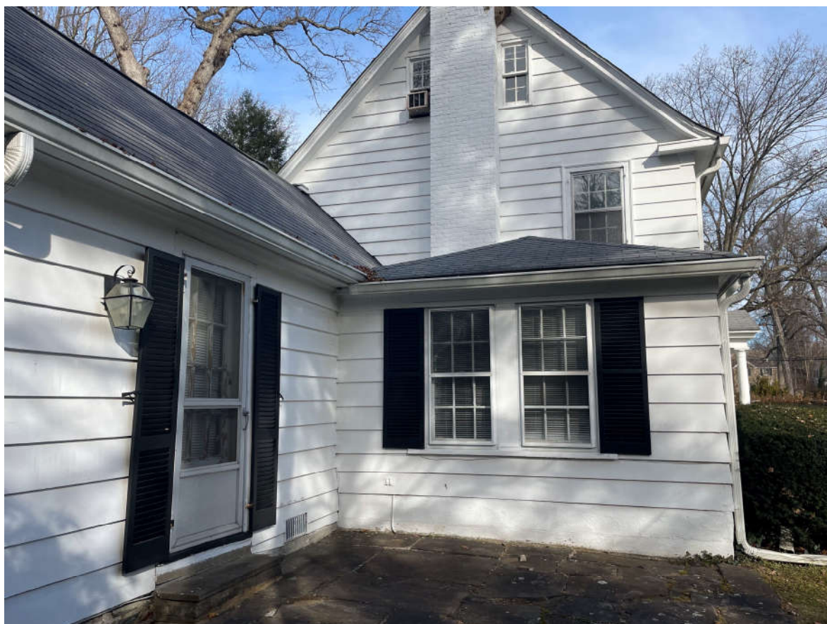
Photo 2: Southwest elevation, former side porch, with 1927 addition at left and main volume at rear, showing junction of roofs and demonstrating later construction of the addition. Photographer: Kyle Toth, M.S., 2023
