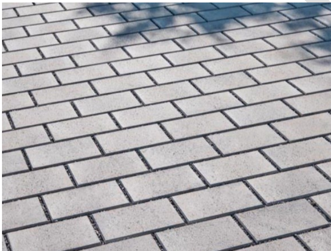
Figure 10: Example of Permeable Pavers
