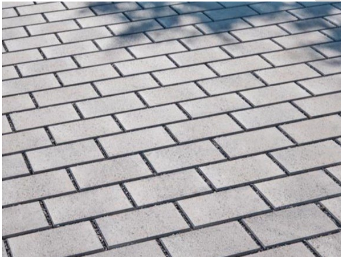
Figure 10: Example of Permeable Pavers
