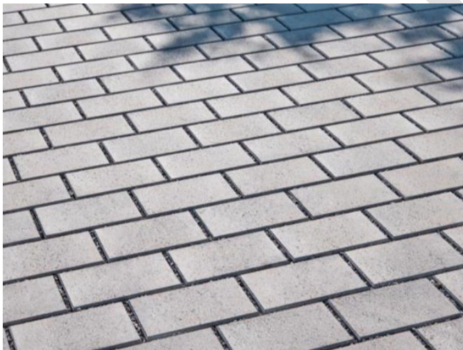
Figure 10: Example of Permeable Pavers
