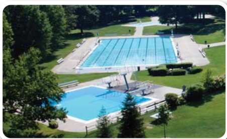
Scarsdale Municipal Pool Complex
