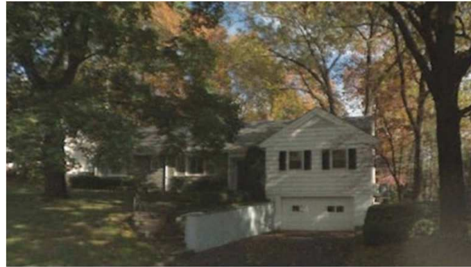
8 Kent Road BEFORE DEMOLITION
